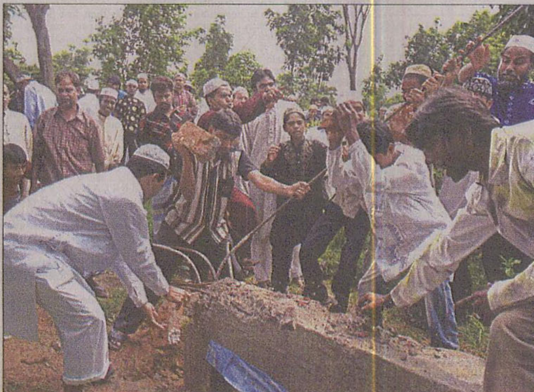
Angered by the Dhaka City Corporation move to construct a road over the graves of their dear ones in Azimpur graveyard, people demolish part of the road after Juma prayers yesterday.
