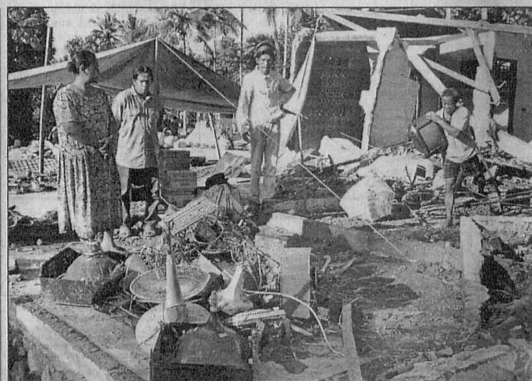
Residents collect their belongings from the ruins of their house in Sinjai, South Sulawesi yesterday, four days after floods and landslides hit six districts. Indonesian rescue workers trawled through remote villages and scoured islands for bodies and survivors from floods and landslides in South Sulawesi as the death toll rose to 216.
