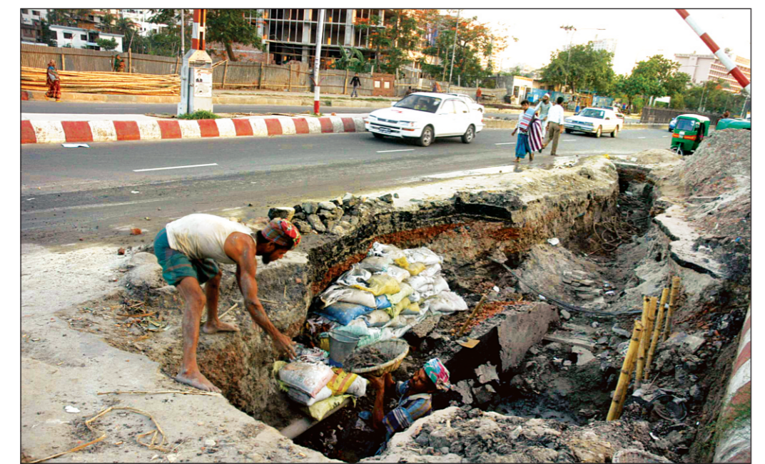
PHOTO: STAR Repair work of underground electricity lines going on for the last two weeks near Karwan Bazar in the capital while the dug up road poses threat of accident.
