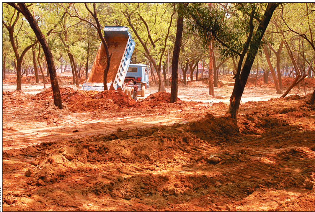
Excavation work for an artificial lake at Osmani Udyan continues.
