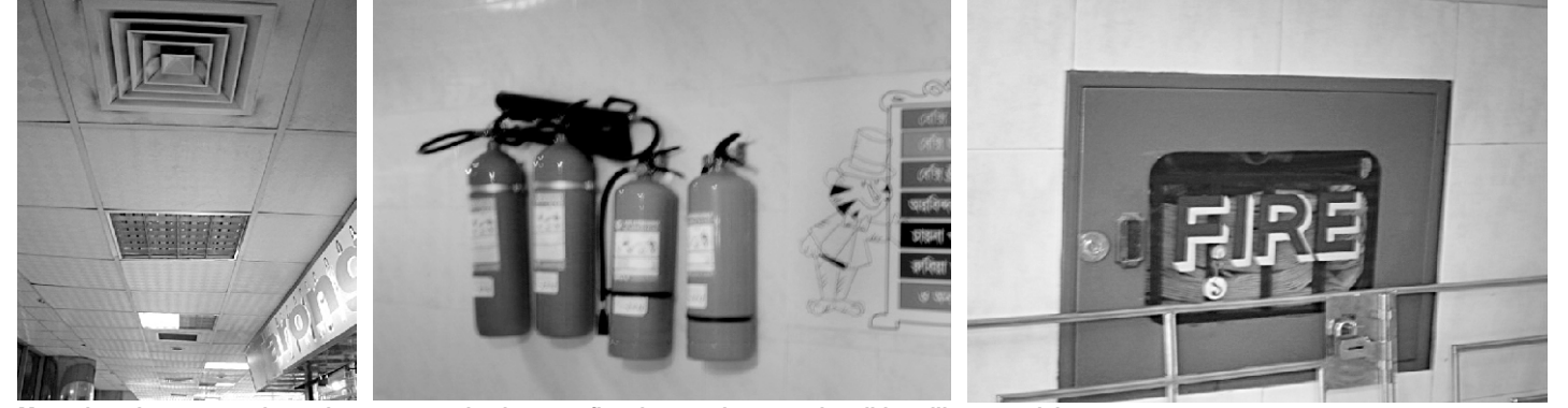
Most shopping centres do not have any smoke detector, fire alarm and use combustible ceiling material.
