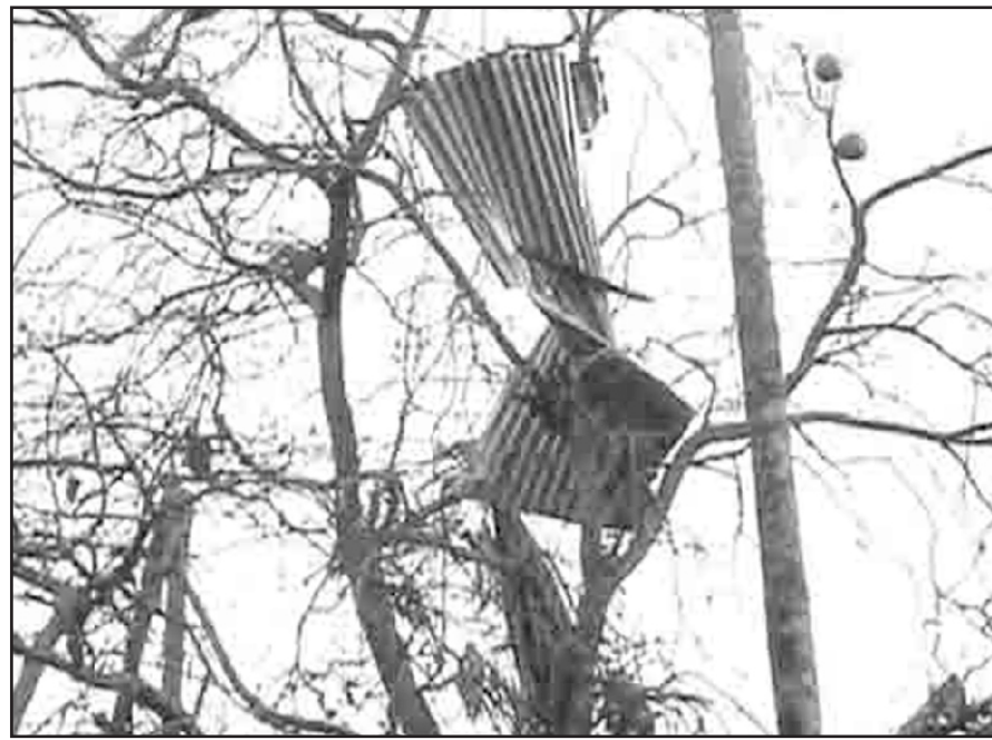
Ablown away CI sheet atop a tree (left) and a tore down house in Karli village in Netrakona Sadar upazila after Tuesday's nor'wester.
