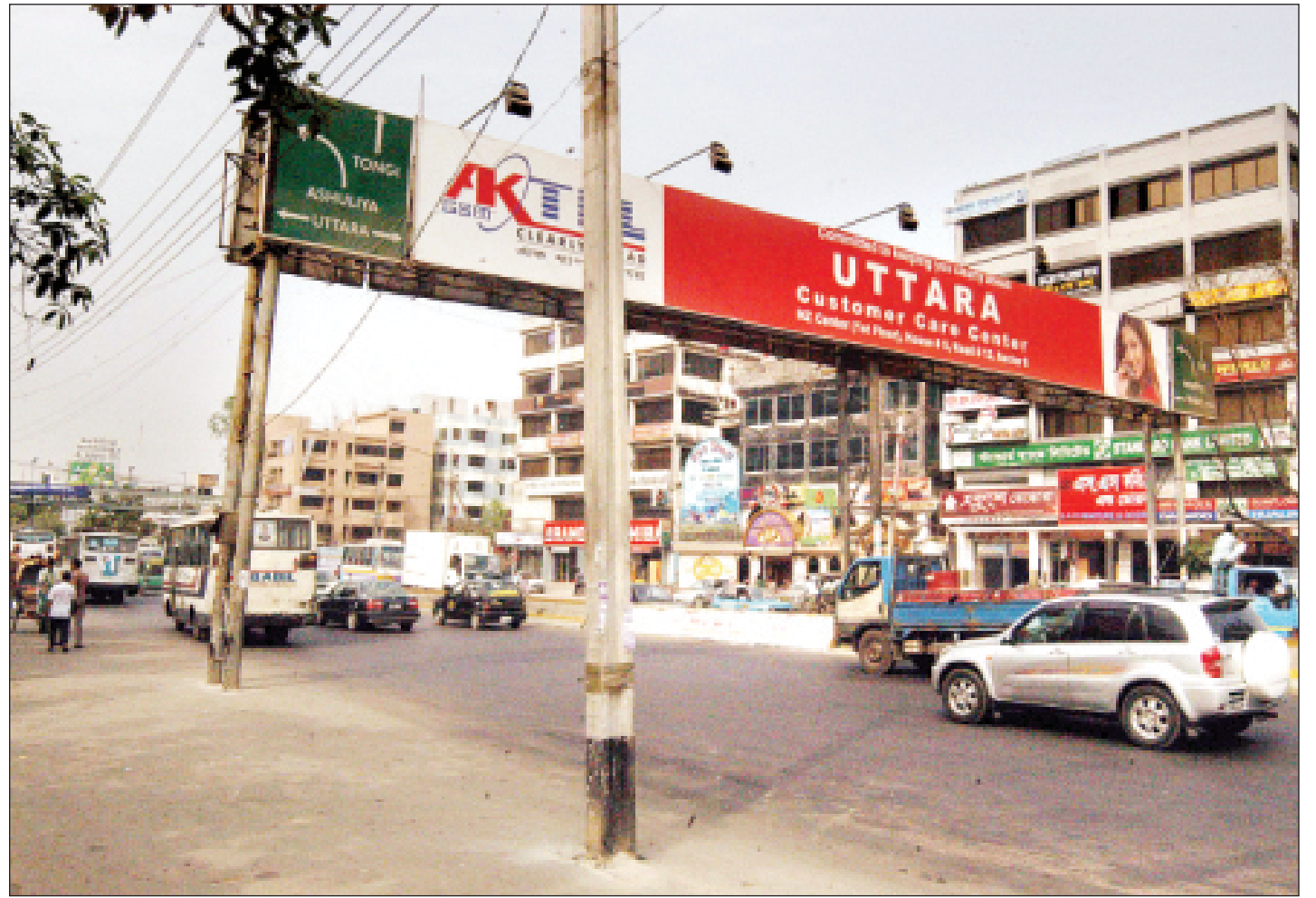
An overhead advertisement arch built illegally on a road in Uttara in the capital.
