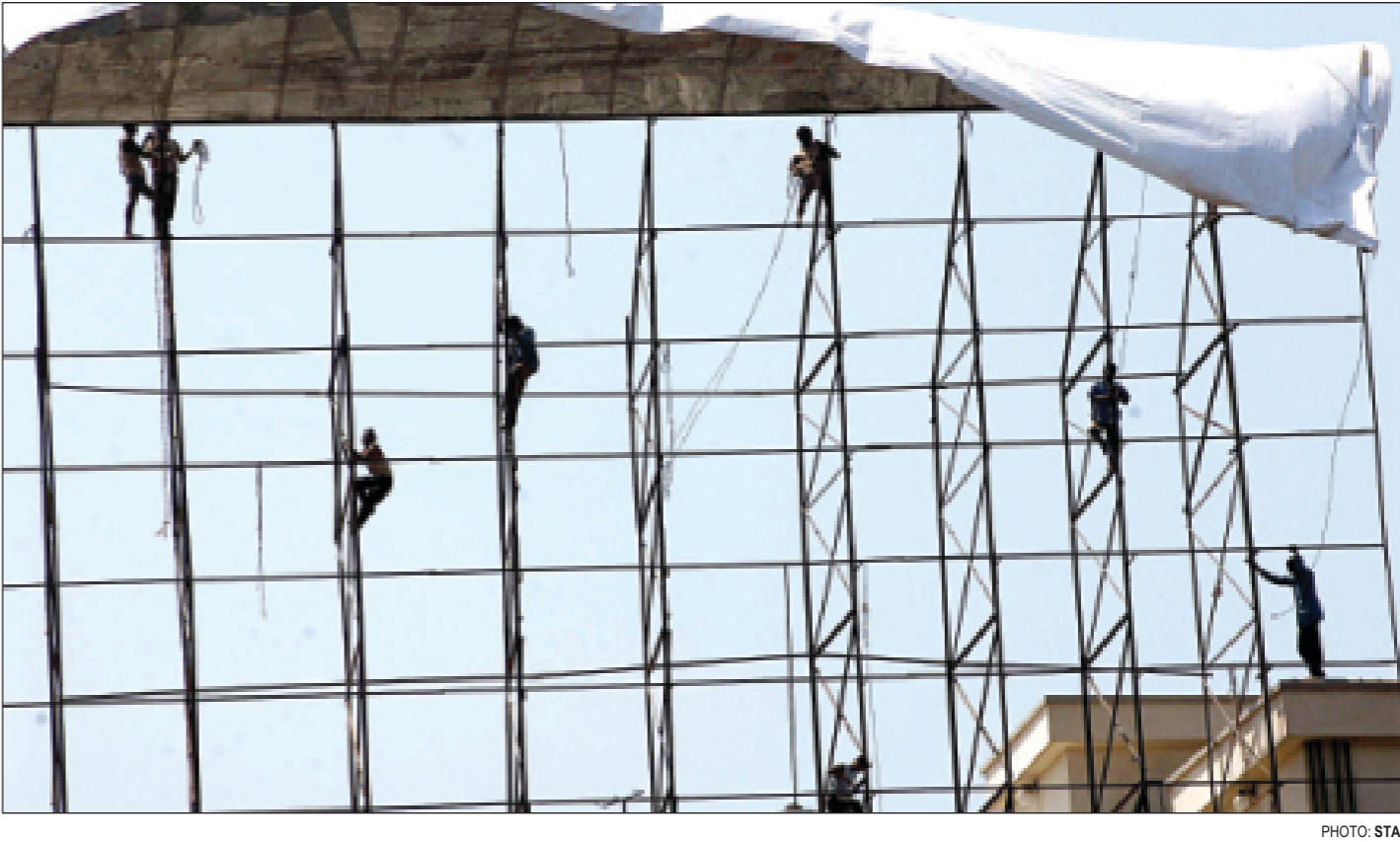
SAFETY SECONDARY... Workers erect a huge billboard on the roof of a building near Asad Gate in the city yesterday with hardly any safety gears on.
