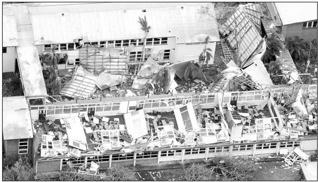
Tropical cyclone Larry crossed the Australian coast near Cowley Beach, south of Cairns yesterday. Picture shows destruction the cyclone caused to the Innisfail High School.
