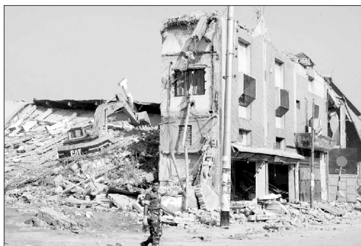
Building collapsed in Tejgaon on Feb 25
