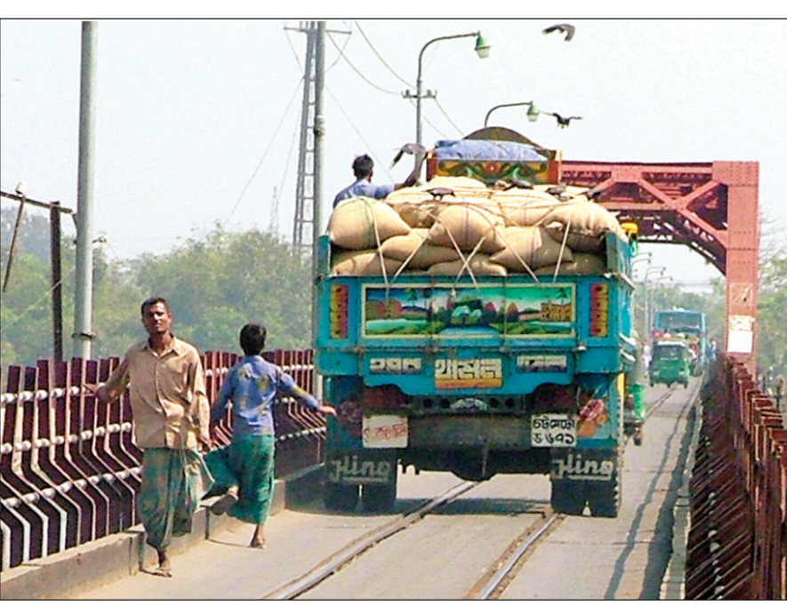
A heavily loaded truck plies through Kalurghat Bridge ignoring weight limit, left, and a woman, right, clenches the railing when a bus runs through the bridge.
