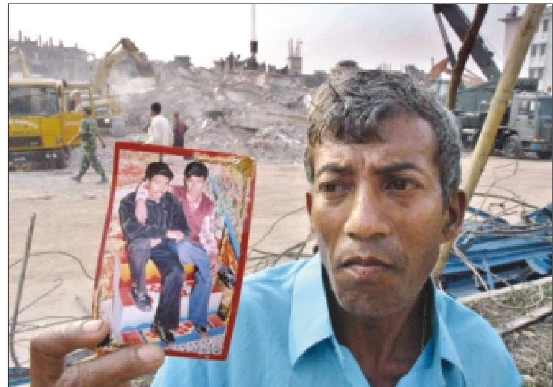
Suranjan, holding a photo of his missing son Nikhil, waits for a miracle at the collapsed Phoenix building in Tejgaon yesterday. Mason Nikhil was working in the building as it tumbled down on Saturday.
