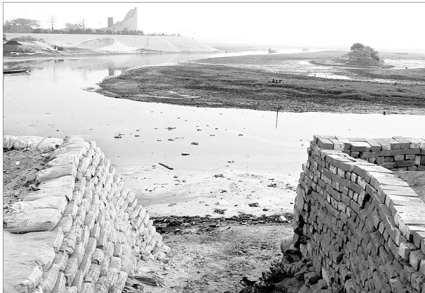
An encroached section of Atir Khal.
