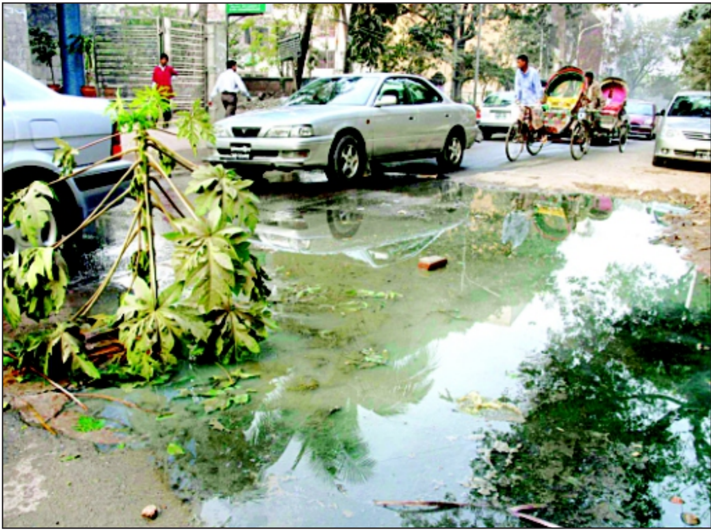
A sewage manhole overflows on Dhanmondi Road-6 in the city, causing suffering to pedestrians as well as passengers. Somebody has also kept a branch of a tree in the open manhole as a sign of warning. The situation continues for nearly a week, but the authorities remain indifferent.
