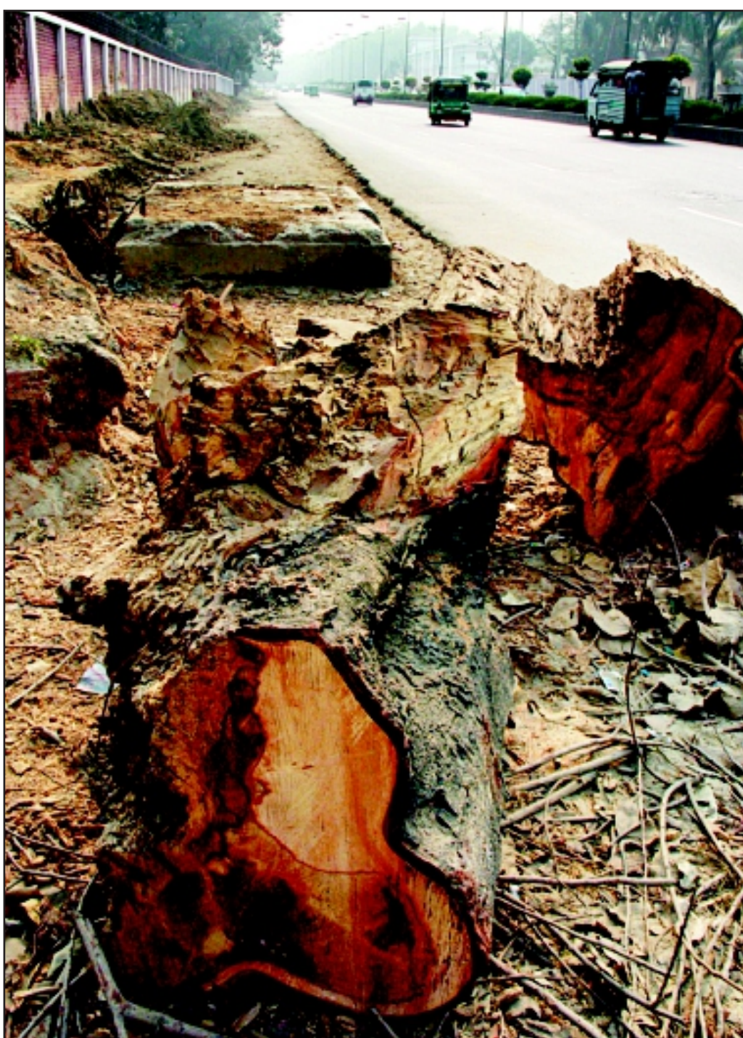
Roadside trees along the stretch of a road from Bijoy Sarani to Banani in the city have been felled as part of a road expansion and development project.
