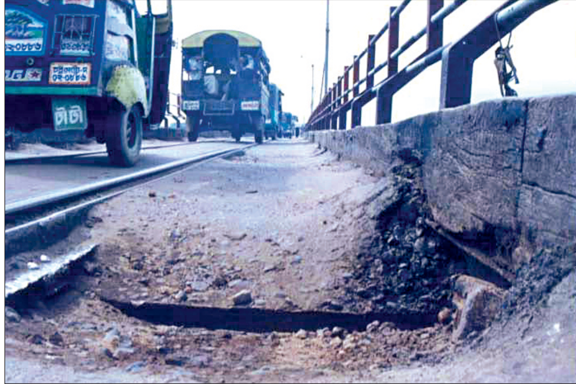
Kalurghat Bridge (Left) has developed several big cracks with huge holes over the years. And despite having rail bits on the entry points of Shah Amanat Bridge (Right) to bar heavy vehicles, they find no difficulty by giving their bodies special shape to cross the bridge risking the lives of passengers.
