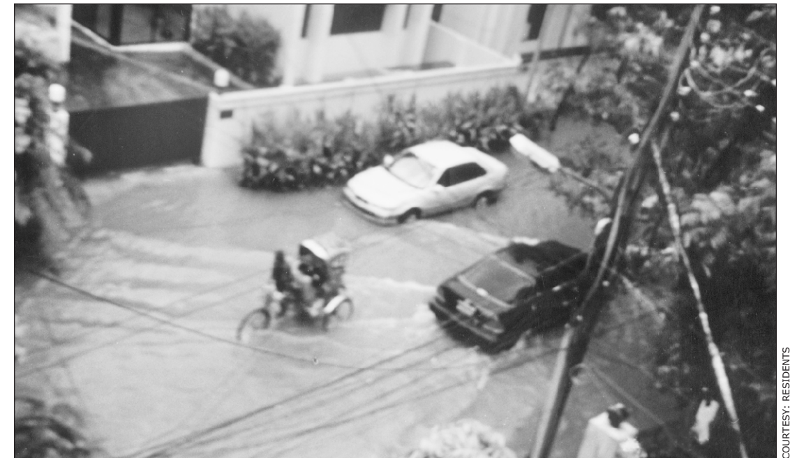
Surface drain water clogs road no 19A. The only conduit into the lake is sealed on an allotted plot of land.
