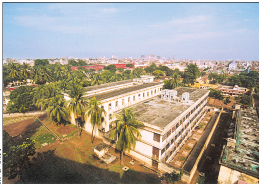
The severely overcrowded Dhaka Central Jail compound in Old Dhaka.
