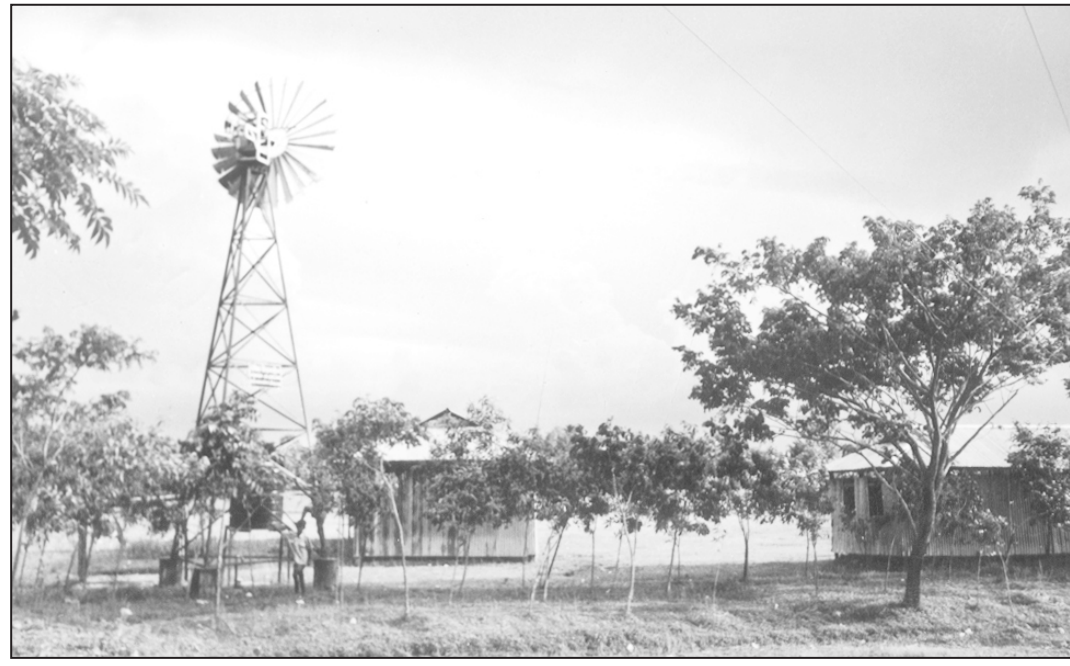
A wind turbine has been installed at Baromari High School in remote Garo hills in Nalitabari upazila, Sherpur for generation of electricity. The Local Government Engineering Department (LGED) installed the wind turbine at a cost of Tk 80,000 and plans more in the area.
