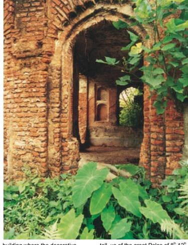
building where the decorative plasters have been peeled off from the brick walls is covered with plain cement plaster without any regard for the original form and shape in such a manner that the building is defaced beyond recognition. Many of the cast iron brackets, lamp fixtures and decorative glazed tiles, which are still visible, are missing every day as time passes away.
