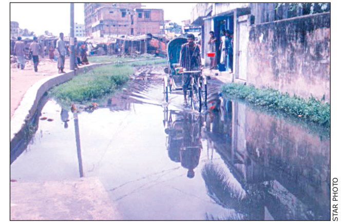
This is a road, not drain though appears so. The Bahaddarhat-Chandgaon link road near the Bahaddarhat market has virtually turned into a drain with sewerage water overflowing into it throughout the year. Not only the commuters, also the residents of the roadside houses suffer a lot. The pedestrians find it difficult to cross the area without getting wet as speeding vehicles create splashes of dirty water. Health hazards are also a cause for concern among the nearby residents, but the authorities have turned a blind eye to their plight. The road also stands testimony to the dilapidated state of the drainage system in the city.
