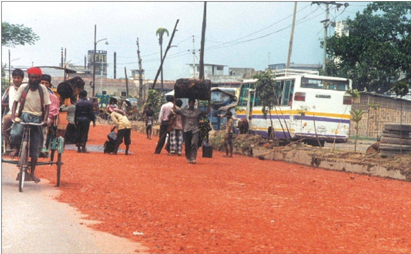
Workers pave the Dhaka-Narayanganj Highway at Shyampur with bricks although the Roads and Highways Department suggests stone layers for all high-ways.
