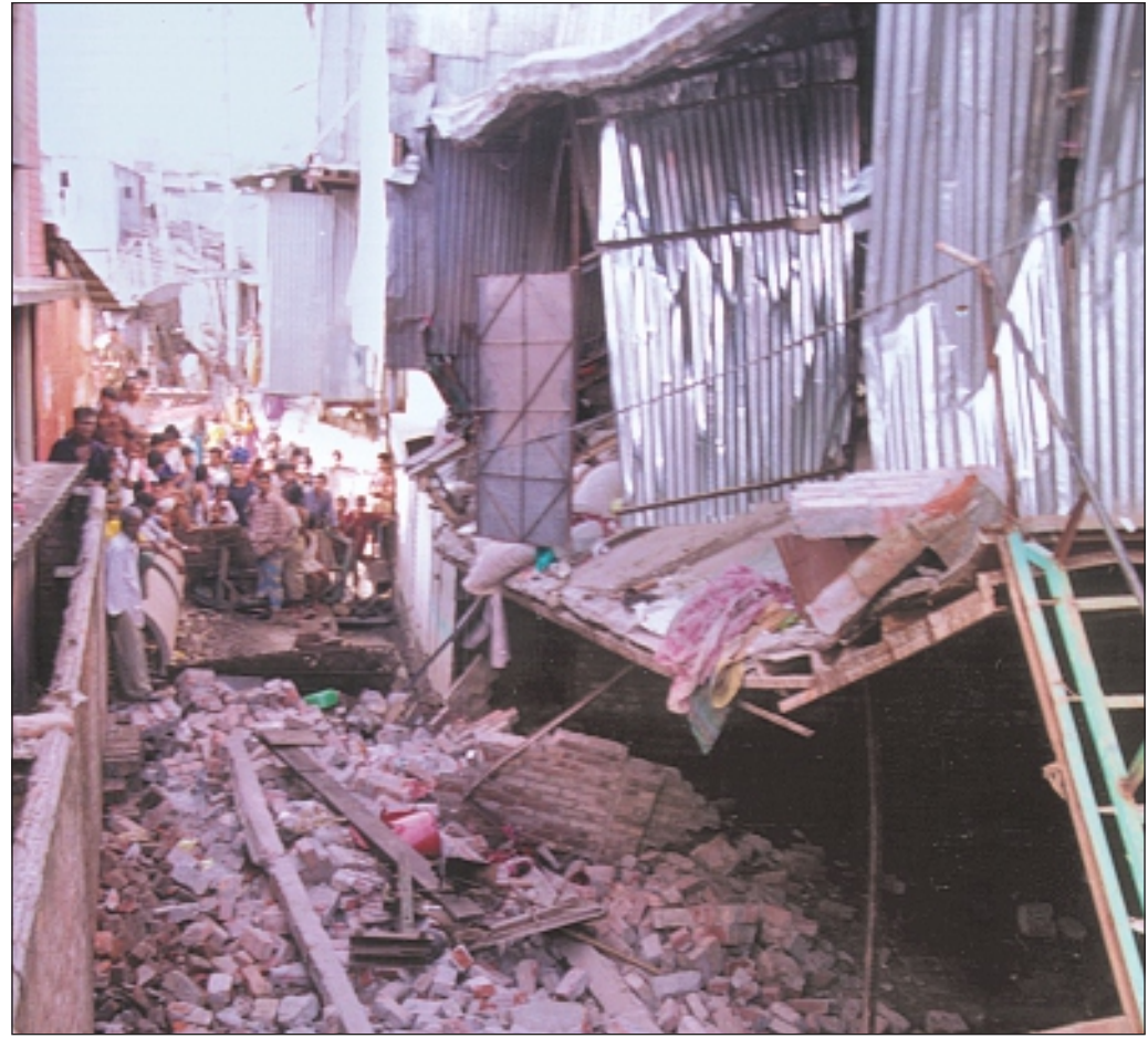
A house collapses in debris in Lalbagh's Rahanganj in the old quarter of Dhaka yesterday, miraculously without any casualty.
