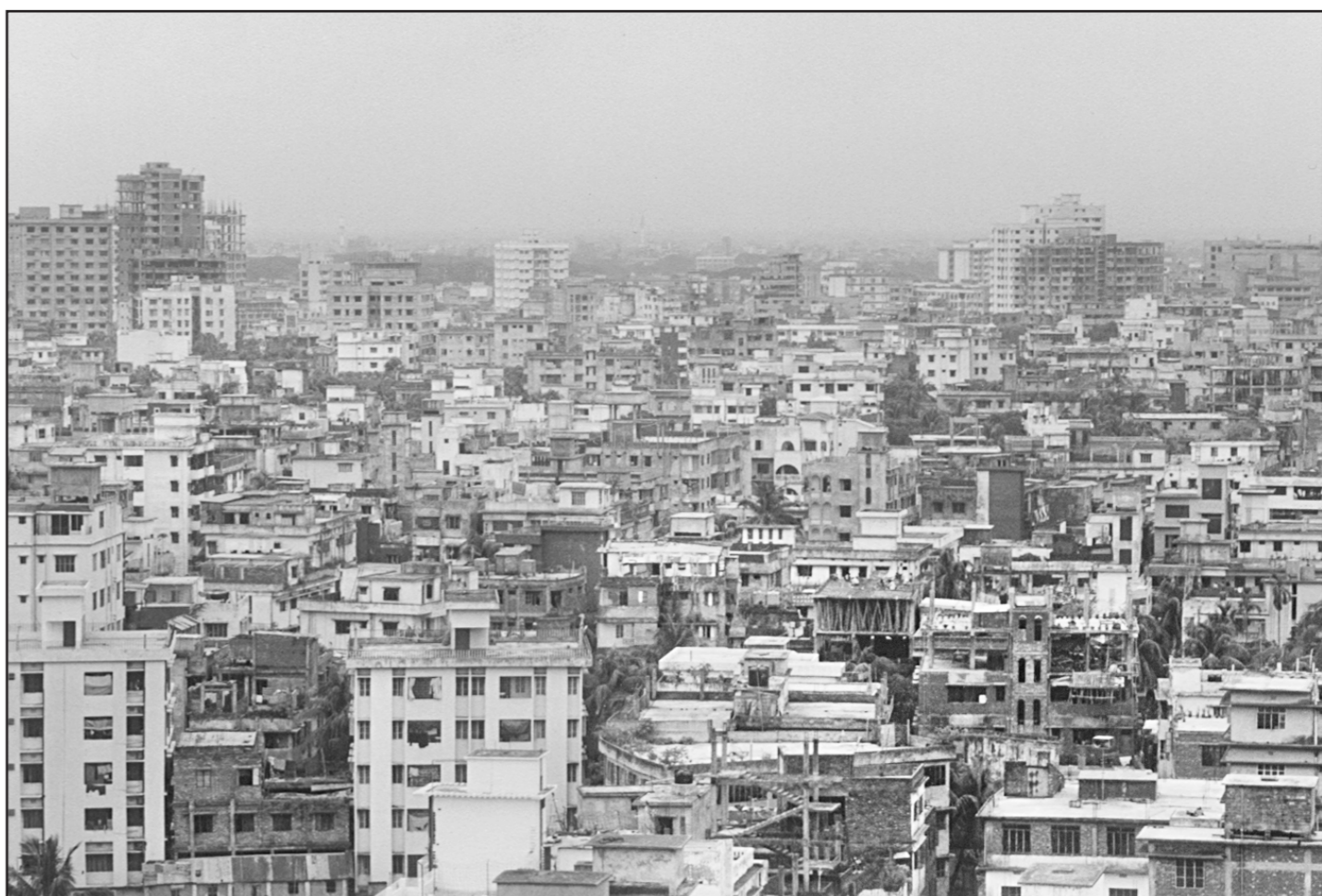
The effect of an earthquake on a building depends basically on its distance from the epicentre, soil type, total weight and structural type and configuration.
