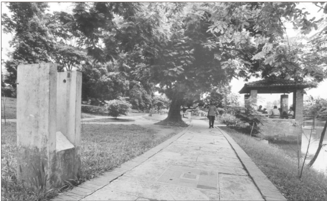
All is set for installing lights along the walkways of Dhanmondi lake. But when will they be lit?
