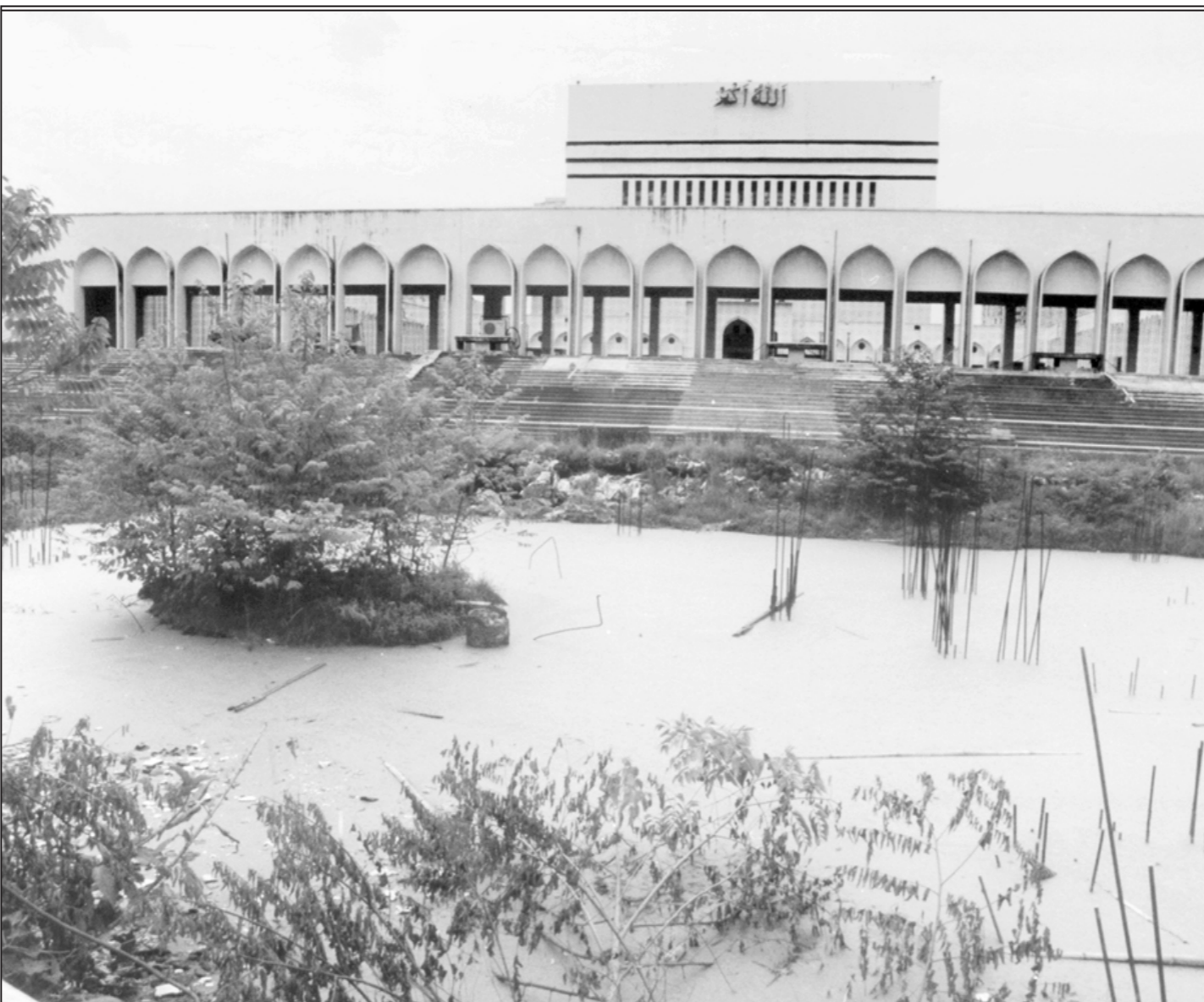
An extension of Baitul Mukarram National Mosque is today a pool of stagnant rainwater and possible breeding ground for mosquitoes. Its construction work began during the immediate past Awami League government.
