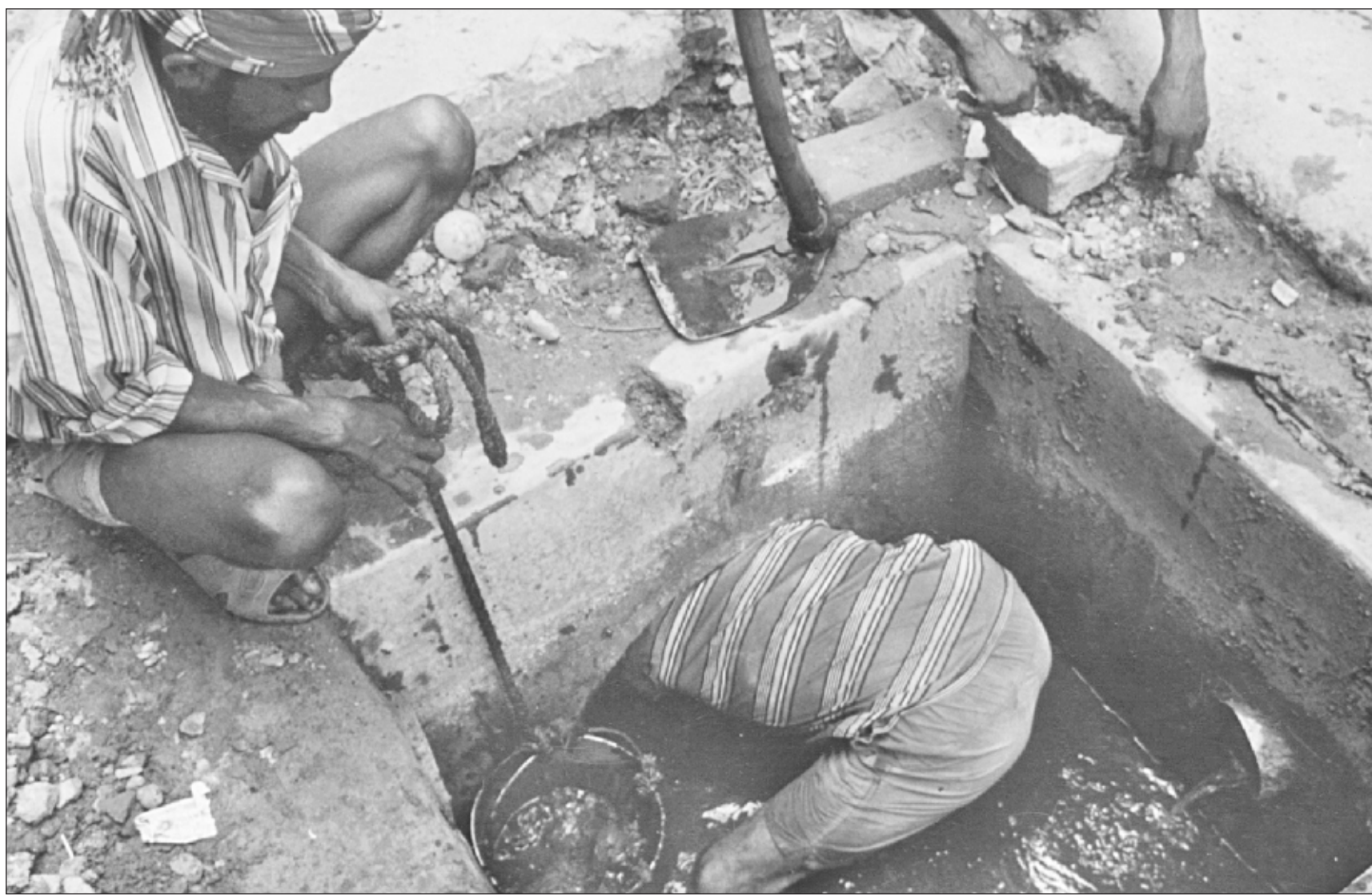
The safety measure is as simple as dropping a lighted matchstick within the tank. If it creates a flame in the reservoir the presence of poisonous gases is confirmed.
