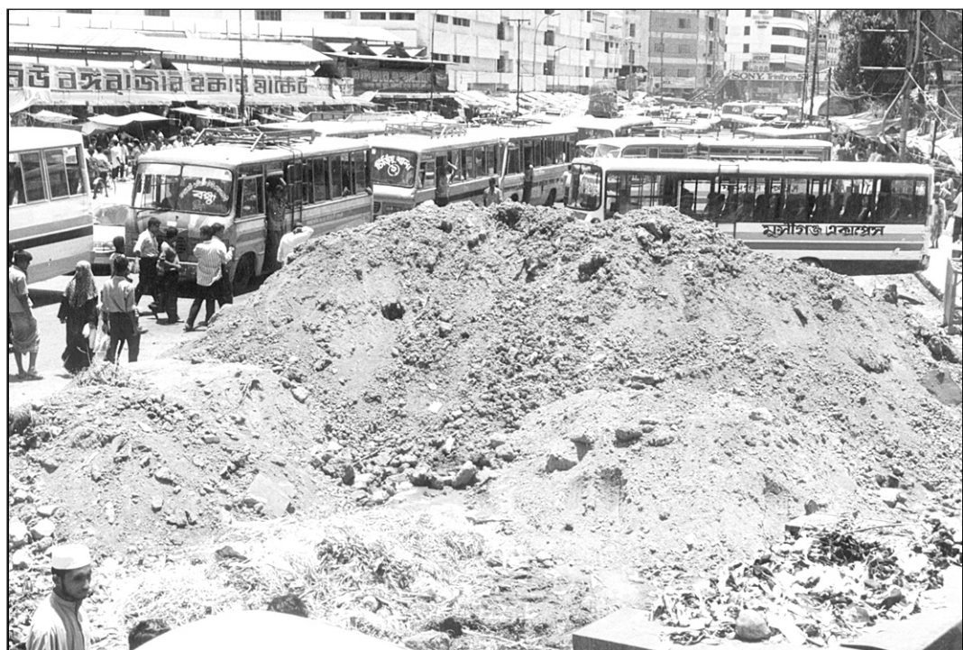
A giant pile of earth on the main road in front of Bangladesh Telegraph and Telephone Board office hinders traffic movement during rush hours, causing sufferings to commuters. Transport operators and commuters on the scene demanded immediate removal of the mound.
