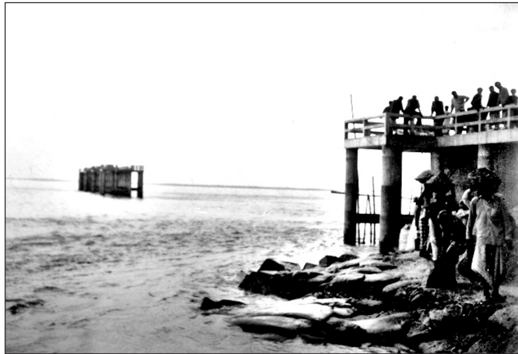
A major portion of a spur in Jamuna river at Shimla in Sirajganj Sadar upazila has been washed away due to heavy rain and onrush of water from the upstream.
