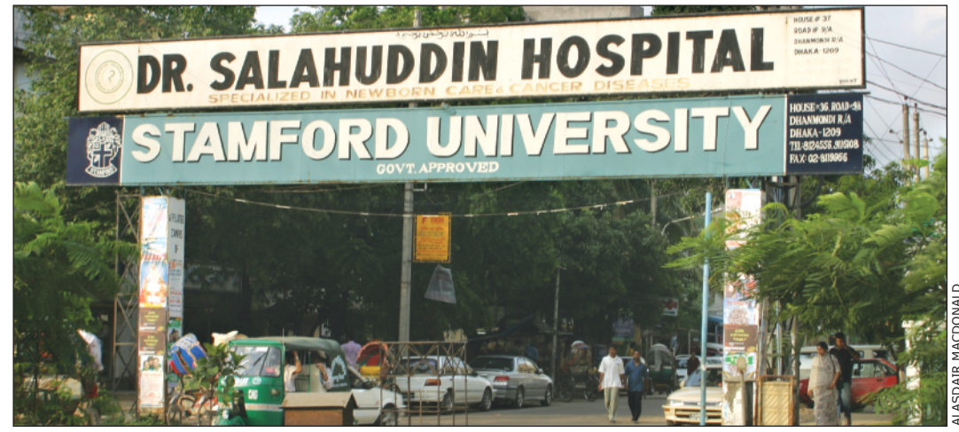
Overhead advertisements like these in Dhanmondi pose threat to public safety.
