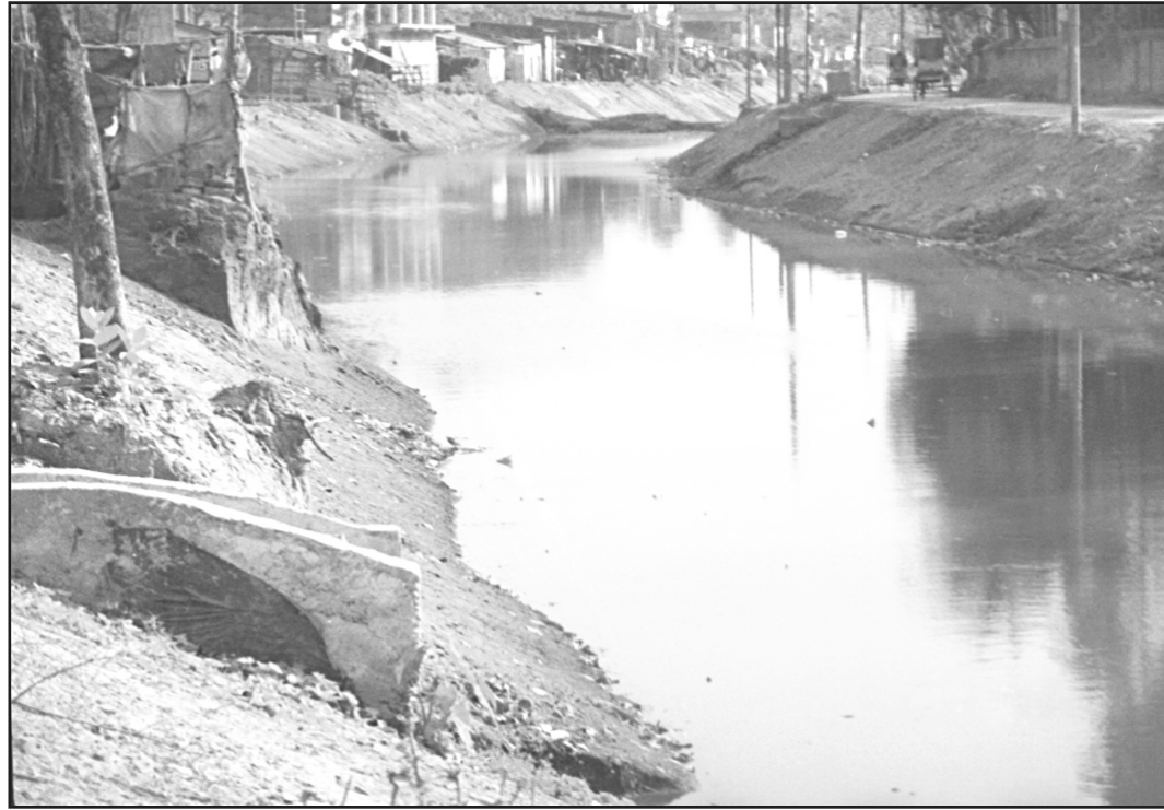
A part of Pranshaher Khal at Satkhira that has been re-excavated.
